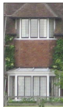
Projecting bay at Westlington House
