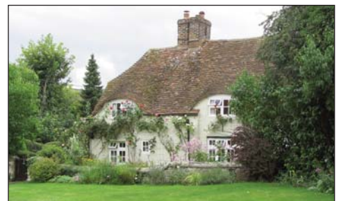
View of field cottage in Upton
