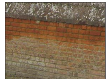
Examples of brick walling
