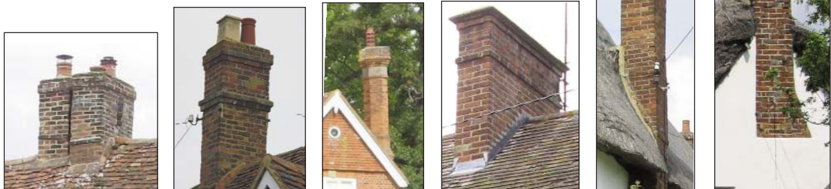
Variety of brick chimneys
