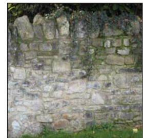
Rubblestone walls in Dinton
