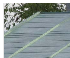
Copper roof at Pinehill
