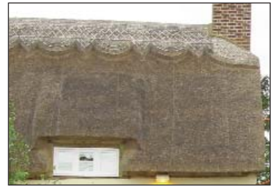
Newly laid thatch
