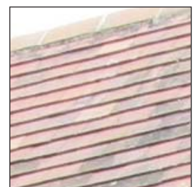
Machine-made clay tile
