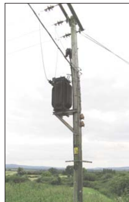
Telegraph pole in Upton
