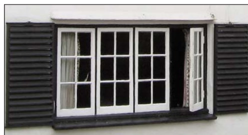
Timber casement with shutters
