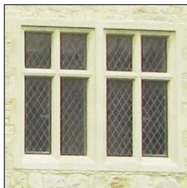
Stone mullions with leaded lights at Dinton Hall
